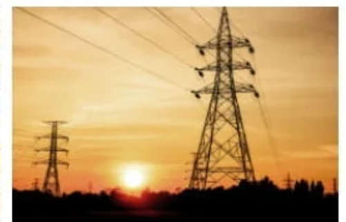
Power Line Inspection
